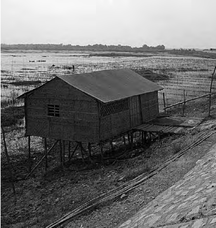
The road was not just expanded but also raised to protect it from flooding during the rainy season, creating problems of access for people living along the road.
