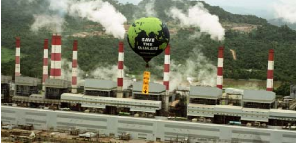
SAVE THE CLIMATE. Greenpeace balloon flies over Mae Moh coal-fired power plant in Lampang, Thailand. Mae Moh Power Plant releases around 1.6 million tons of sulfur gas everyday and more than four million tons of carbon dioxide emission in the atmosphere annually. Around 200 have died due to lung cancer and respiratory diseases since it started operation. (Photo by Greenpeace/Unanongrak)
