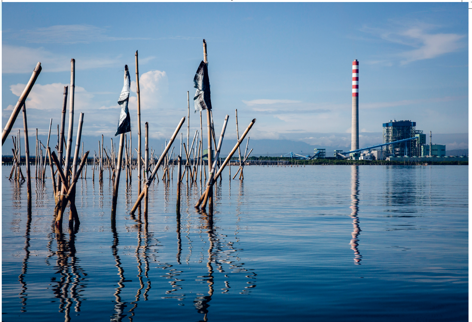
Cirebon is a fishing village in Indonesia whose residents are engaged in fishing, salt farming and agriculture. Since the Cirebon coal-fired power plant was built, their lives have changed. As pollutants from the coal power plant contaminated the water and killed many marine creatures, fishers lost their livelihood. Air pollutants caused a spike in lung and heart disease. © Ulet Ifansasti / Greenpeace (2.5.2019)
