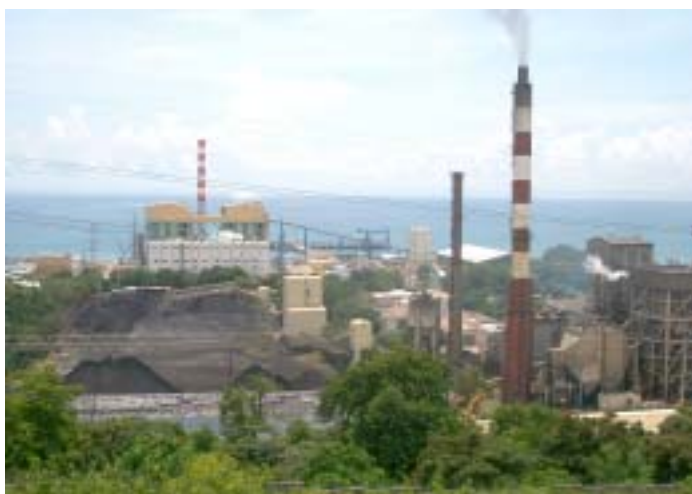
THE VIEW. The ADB-funded 200-MW coal power plant in Cebu, Philippines.
