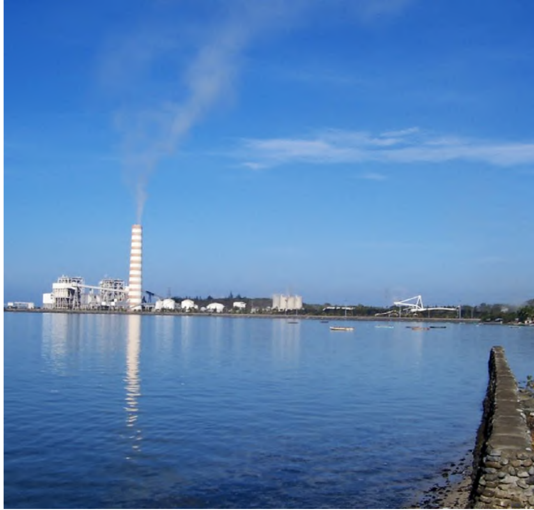
Masinloc Coal-Fired Power Plant
