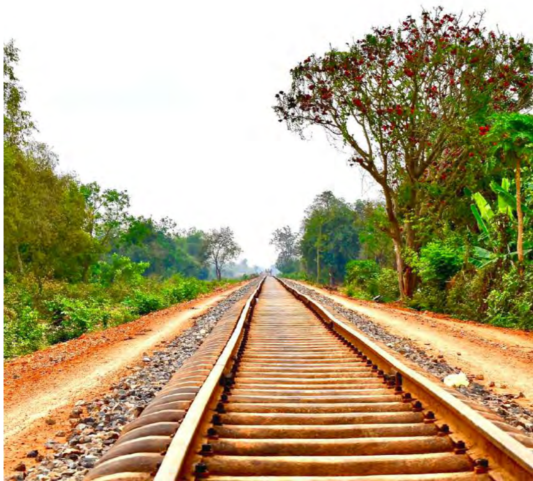
GMS Rehabilitation of the Railway in Cambodia
