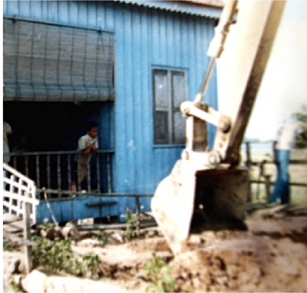
Phnom Penh to Ho Chi Minh City Highway Project
