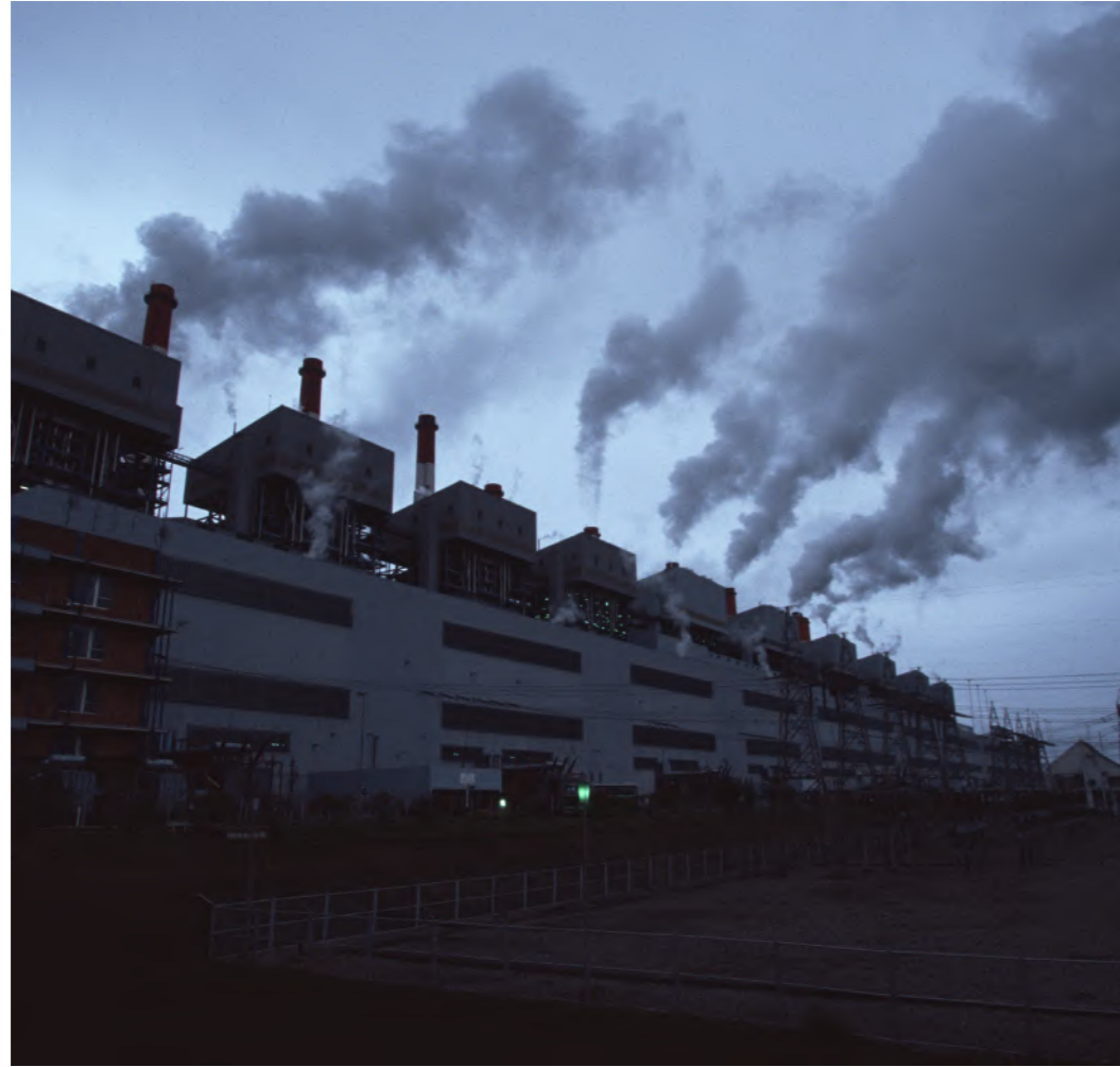
Mae Moh Power Station
