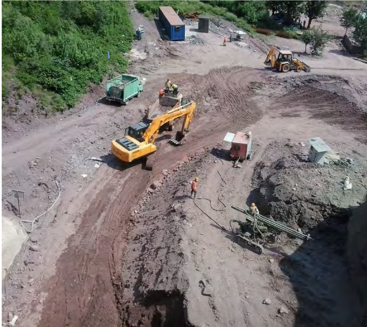
This page | The ongoing construction of the Kiratpur Ner Chowk Expressway
