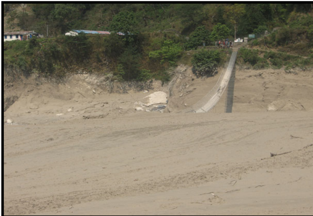
Seti fury: collapse of hanging bridge after May 2012 flood, Photo credit: Kantipur daily
