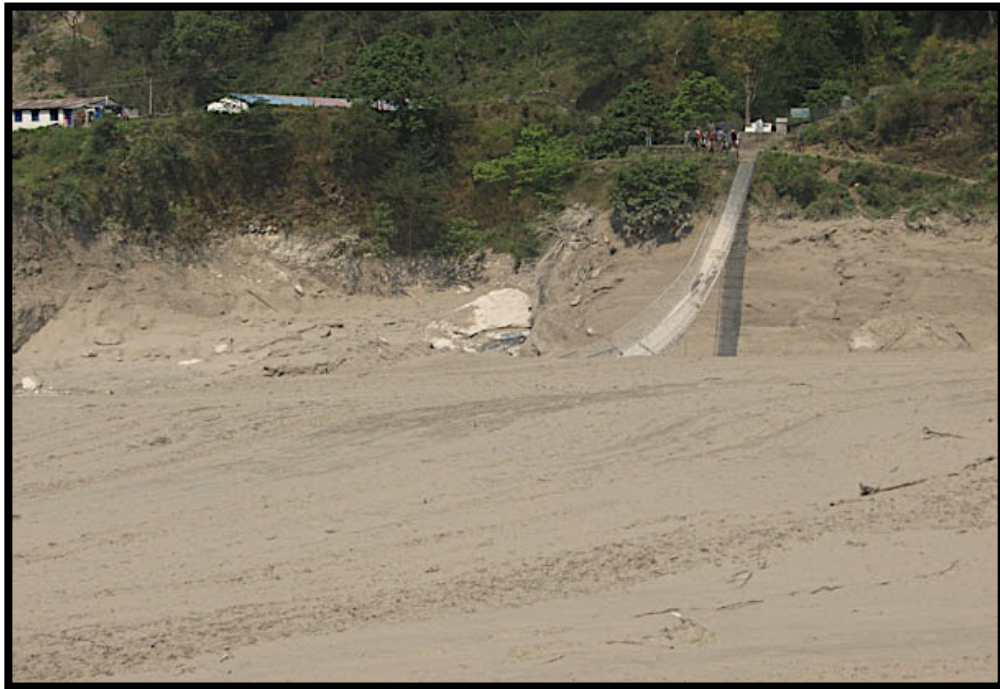
Suspension bridge after Seti flood in 5 May 2012, Photo credit: Kantipur daily
